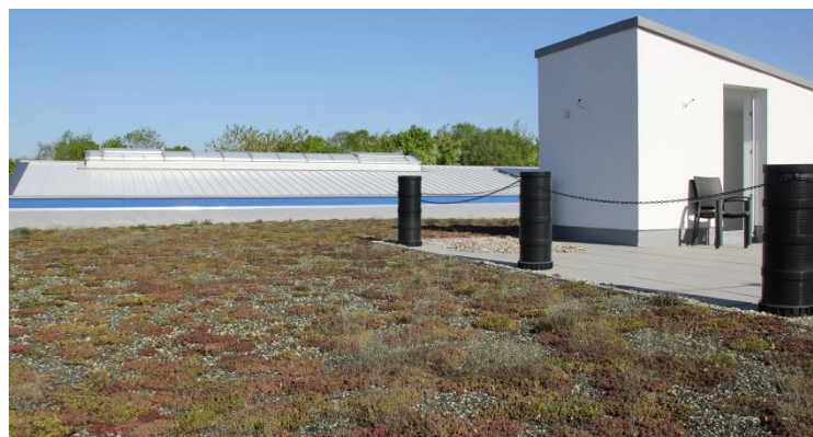
Picture 5: Green roof on top of the main building
