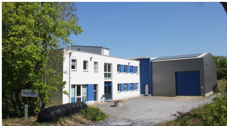
Picture 1: INTEWA company building
