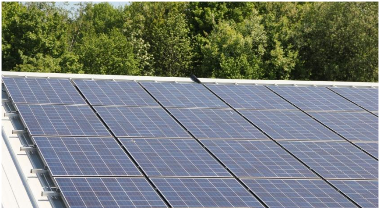
Picture 7: Solar system on the hall roof
